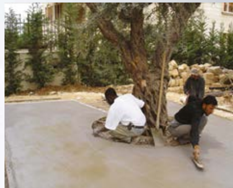
4- Float and the trowel the surface of the fresh colored concrete.
