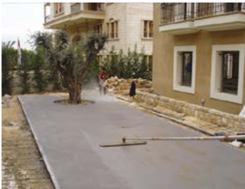
3- Color Hardener should be well spread by bull-floating it.
