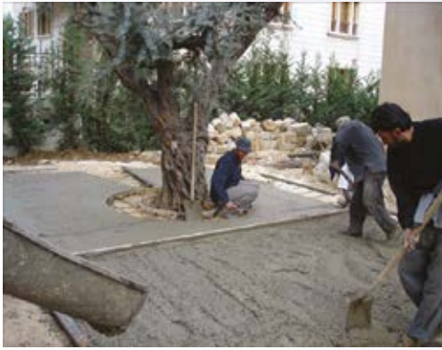
1- Ready-Mix delivered on site
