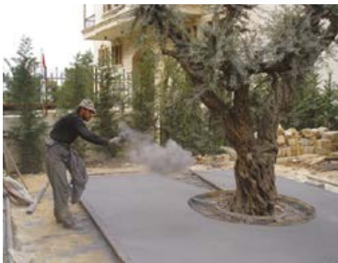
5- Applying Release powder.
